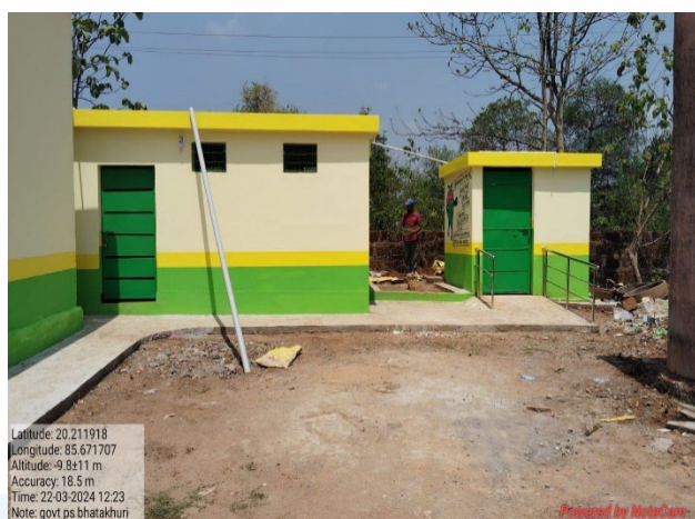
Renovated toilets in 2 schools in Jatni, Khordha
