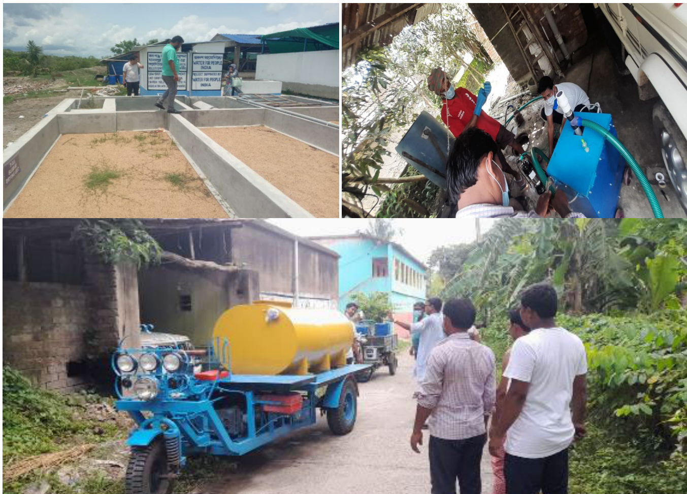
Faecal Sludge Treatment Plant set-up; Demonstration of sludge collection; Assembled Cesspool
